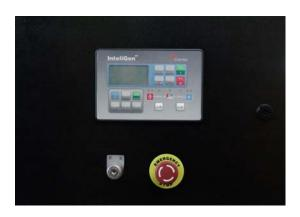
Automatic Parallel Control Panel This new automatic parallel system adopts intelligent modules, inserted and folded installed, no need the peripheral relay and logic circuit. The main switch adopts electronic breaker or frame breaker, combined together with the generator, which is very reliable. One generator, one panel. The panel can be used both for singly and parallel. It is only need to parallel generator with such panel when the capability needs to be enlarged in the future.
