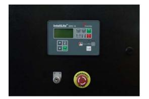
Auto Module Control Panel is the configuration for nobody on duty controlling generators. This kind of panel adopts auto module control system, with large LCD display to show the menu.
